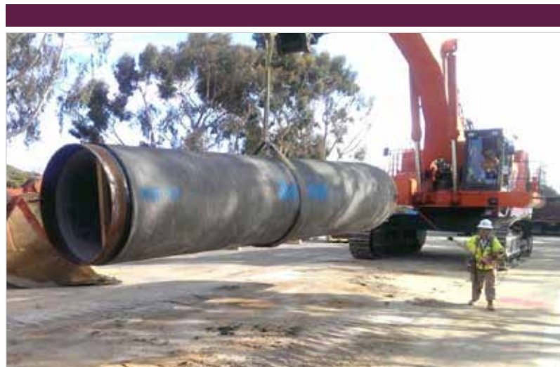
Work crews install a section of 54-inch steel pipe connecting the Lewis Carlsbad Desalination Plant to the Water Authority's aqueduct system.
