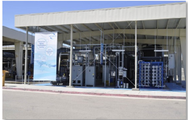
Completed Demonstration Project Improvements in City of San Diego, Proposition 50 Project: Recycled Water Distribution System Expansion and Parklands Retrofit, and Indirect Potable Reuse/Reservoir Augmentation Demonstration Project
