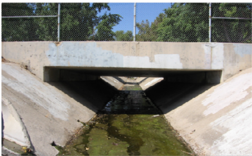
Concrete Channel in Woodglen Vista Creek, Proposition 84 Project: Pilot Concrete Channel Infiltration Project
