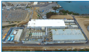
Carlsbad Seawater Desalination $1 billion
