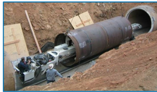
Pipeline Relining $493 million
