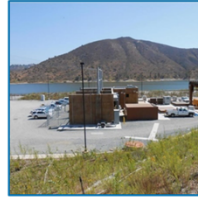
Lake Hodges Hydroelectric and Pump Station Facility $208 million
