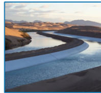
All-American & Coachella Canal Lining Project $447 million ($190 million from Water Authority)
