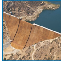
San Vicente Dam Raise & Related Projects $811 million
