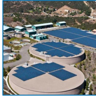
Twin Oaks Valley Water Treatment Plant $179 million
