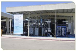
The Water Purification Demonstration Project is evaluating the feasibility of indirect potable reuse/reservoir augmentation.
