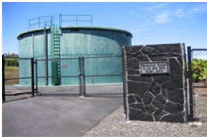
Aging storage tanks can lead to contamination of rural water supplies.
