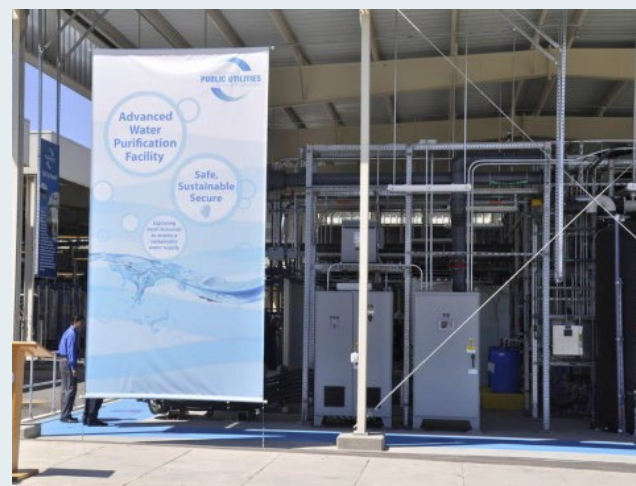
The City of San Diego Advanced Water Purification Facility is conducting pilot testing for indirect potable reuse.
