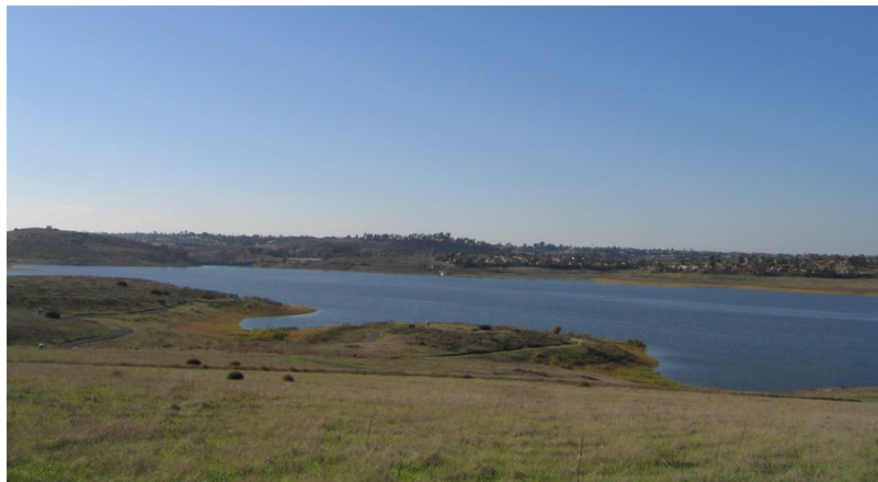
Sweetwater Reservoir, owned by the Sweetwater Authority, stores natural runoff.
