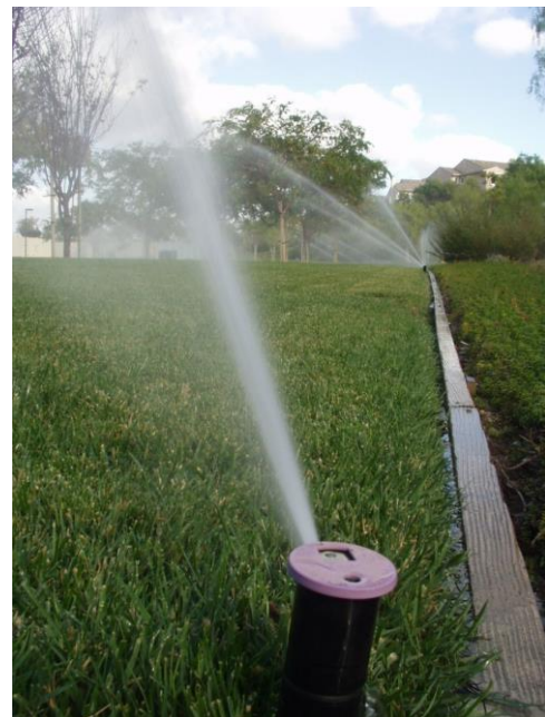
The North San Diego County Regional Recycled Water Project – funded by Proposition 84-Round 1 and Round 2 – features multiple partnerships, watersheds, and beneficial uses.
