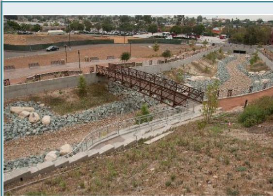
Photo Credit: Jacobs Center for Neighborhood Innovation
