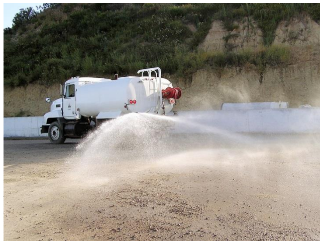
Recycled water is used for dust control at construction sites because drinking water quality is unnecessary.
