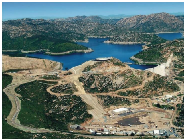
The San Vicente Dam Raise (completed in 2014) will contribute to long-term water supply reliability for the region.
