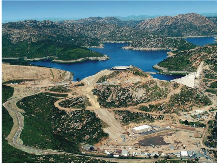
The San Vicente Dam Raise (completed in 2014) will contribute to long-term water supply reliability for the region.
