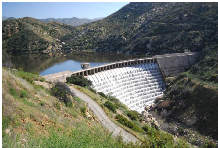
Barrett Dam, shown releasing water, stores surface water in the upper portion of the Tijuana Watershed.
