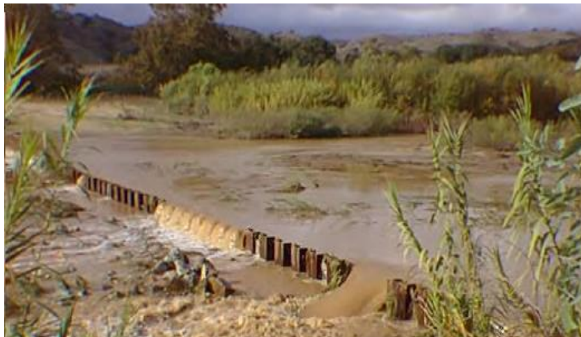
The Santa Margarita Conjunctive Use Project – funding by Proposition 50 – provides for enhanced recharge and recovery from the groundwater basin to provide a water supply for both Camp Pendleton and Fallbrook as resolution of a long-standing water rights dispute with input from the United States Bureau of Reclamation.
