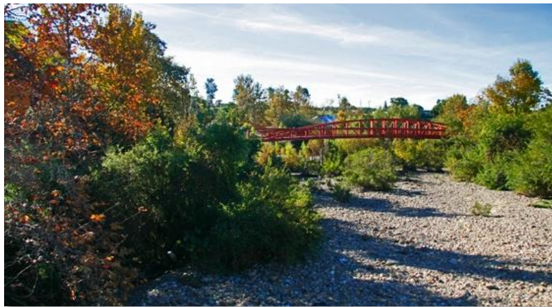
The Chollas Creek Integration Project – funded by Proposition 84-Round 1 – will reduce flooding and improve water quality along Chollas Creek.
