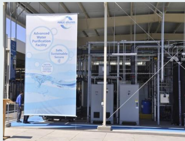
The City of San Diego Advanced Water Purification Facility is conducting pilot testing for indirect potable reuse.
