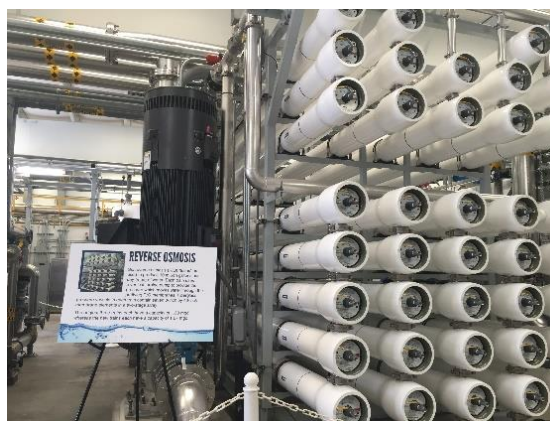
Reynolds Desalination Facility
