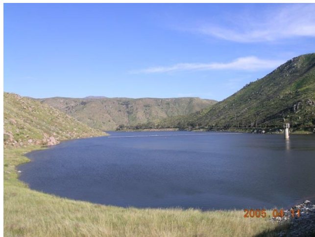
El Capitan Reservoir has a storage capacity of 112,800 acre-feet and holds both surface runoff and imported water.
