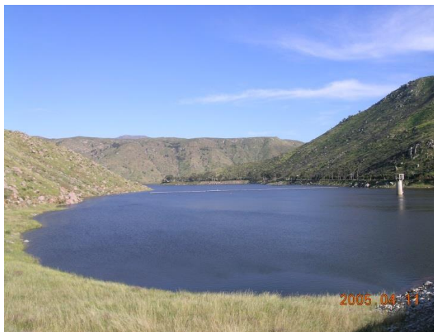
El Capitan Reservoir has a storage capacity of 112,800 acre-feet and holds both surface runoff and imported water. Photo credit: Jeff Pasek, City of San Diego
