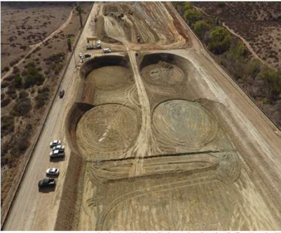
East County AWP Project, Site Preparation – Secondary Clarifier, November 2022
