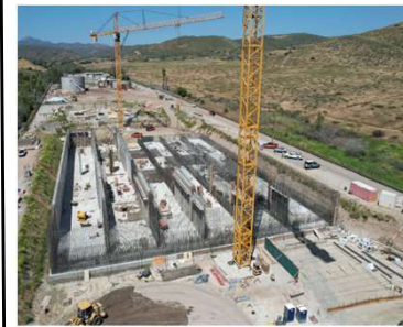
East County AWP Project, Concrete Foundation and Walls – Aeration Basins, May
