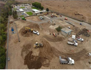
East County AWP Project, Site Preparation – Digesters, October 2022
