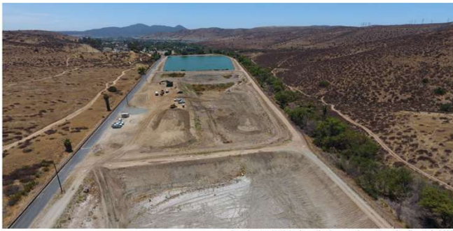
East County AWP Project, Site Preparation – Mass Grading, July 2022
