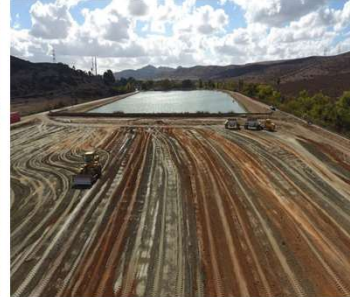
East County AWP Project, Site Preparation – Mass Grading, November 2022
