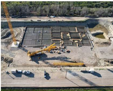
East County AWP Project, Concrete Foundation – Aeration Basins, February
